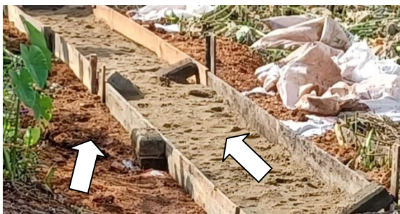
Figure 5. Soil compaction as pathway foundation with sawdust and sand.
