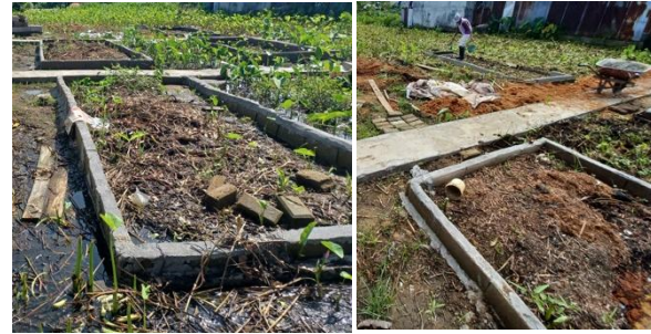
Figure 7. Long-arranged planting area.
