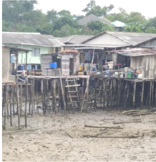
Figure 2. The Condition of Non Permanent Houses on Lengkang Island
