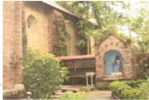
Plate 4. Support buttresses on the right side of the church where grass, algae and moss thrive on its outer face. Also shown is the area for grotto and candle lighting area for parishioners.
