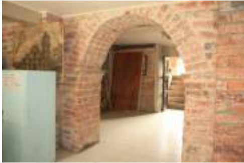
Plate 11. The arched brickwork entrance's keystone had been covered by the recent addition of ceiling. The original clay fired floor tiles have been replaced by modern ceramic tiles.
