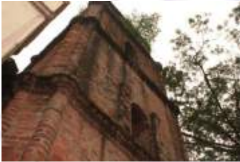
Plate 1. The four-tiered belltower as photographed from the ground with a tree and its roots clinging to the crevices of the brickwork.
