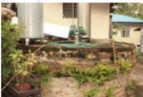
Plate 13. The old well ( bubon ) at the left side of the church, now covered with concrete slab and topped with electric water pumps, steel tanks cylinders and electrical wires.
