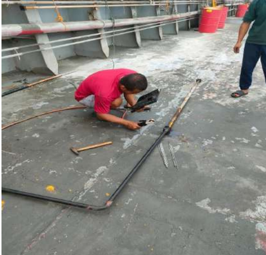
Gambar 3 Proses Perbaikan Metode Flush Welded Patch
