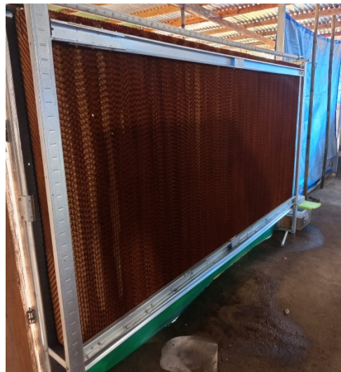
(B). Cooling Pad.
