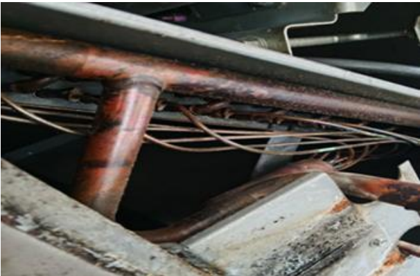
Gambar 5. Evaporator coil Unit Indoor
